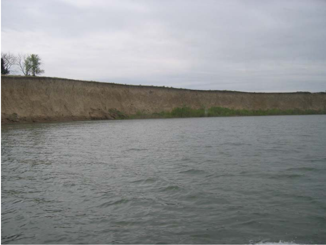
Figure 5 - Large areas of erosion occurring above normal reservoir water surface, elevation 2,366.
